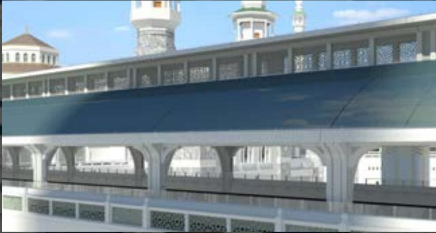
The bridges were designed with arched roofs. The architects wanted the glass in the roofs to have the same domed shape. SUNOVATION was able to meet this specification thanks to silicone encapsulation technology.
